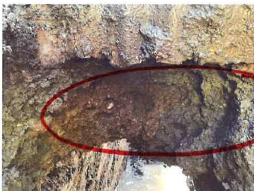
culvert is squished and bottom is deteriorated
