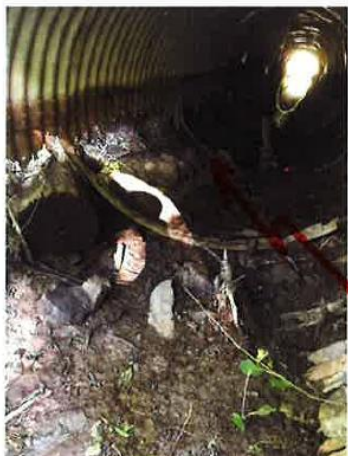
culvert is squished and bottom is deteriorated
